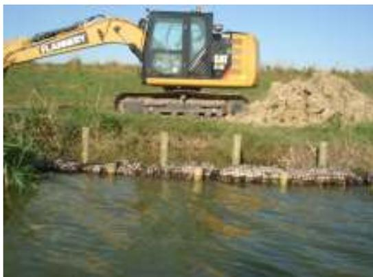
Some of the bank at Piddinghoe being reinforced. Posts are driven in then bags of stone in heavy duty netting are placed between posts. Coir rolls, made from coconut hair are located behind the stones. They are robust and once saturated are ideal for reeds to grow in and get established. The bank is then filled behind and turfed or matting placed to reinforce the bank.
